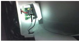
Remove (2)  $11/32^{nd}$  nuts and drop the bottom of the assembly so you can clean excessive grease from underneath the vault door then plug in sensor and power up.
